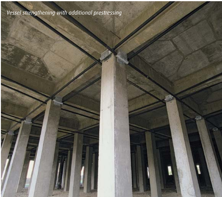
Water tower strengthening with additional prestressing loops
